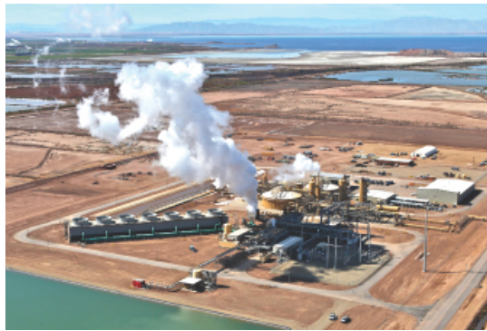
Hudson Ranch Geothermal Project co-developed and financed by Hannon Armstrong
